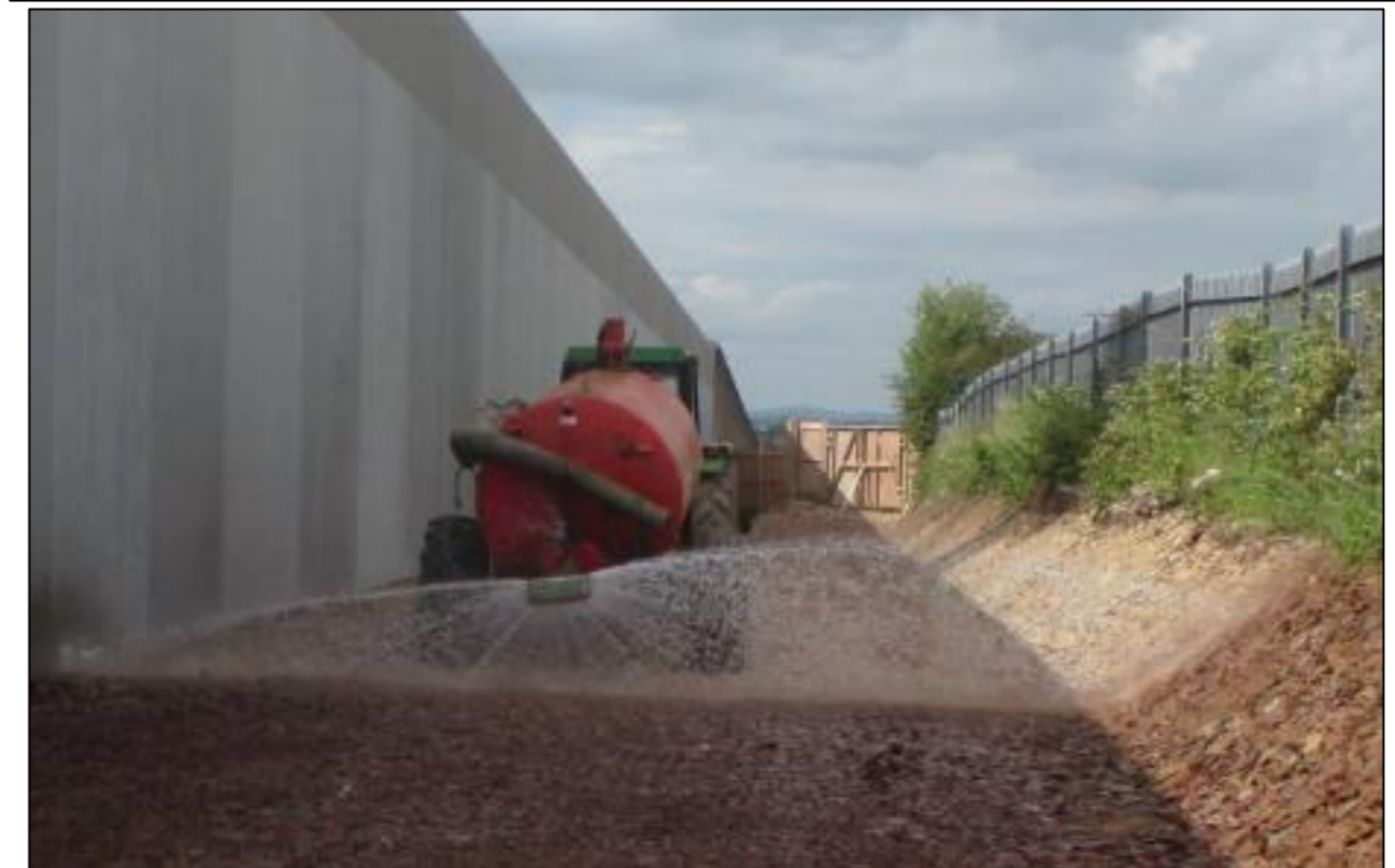
Road Sweeping & Dust Suppression
